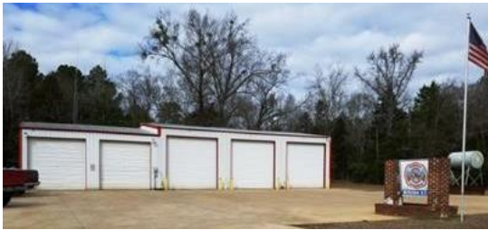
Figure 136: Winona VFD, Station 2
